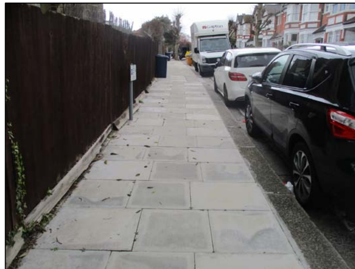
CASE STUDY: NETHERFIELD ROAD, N12
